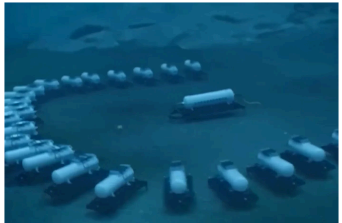
A HiCloud visualization of submerged data center pods arranged in an arc on the ocean floor, illustrating its modular subsea deployment off China's coast.
