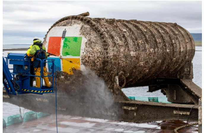
A worker pressure-washes barnacles and algae from the recovered Natick pod, revealing the Microsoft logo beneath two years of biofouling.
